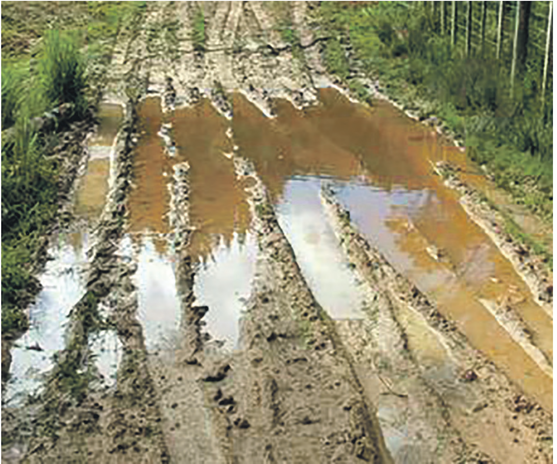
Adequate drainage when building a laneway or track is paramount.
