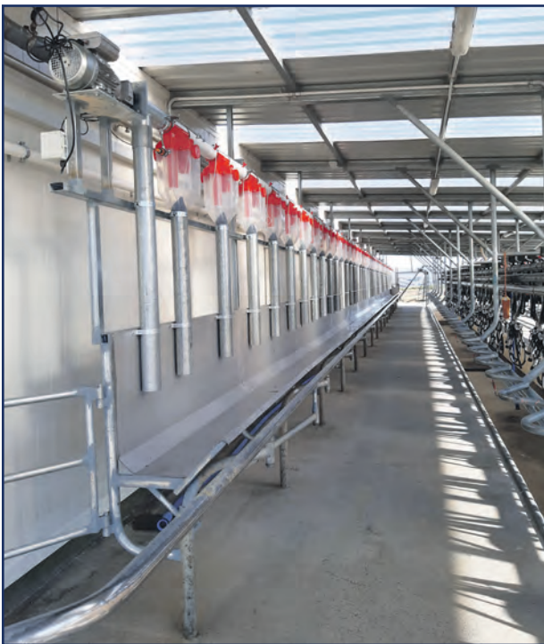
In-shed feed system install, herringbone and rotary.
