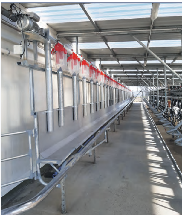
In-shed feed system install, herringbone and rotary.
